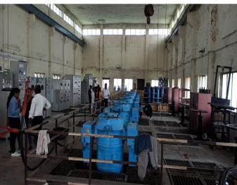
Mr.Ganesh Dhaware had given guidance about how to water distributed by Power control panel with six 600 hp induction motor are used. He explained the working of induction motors and controlling the motors using power panels
